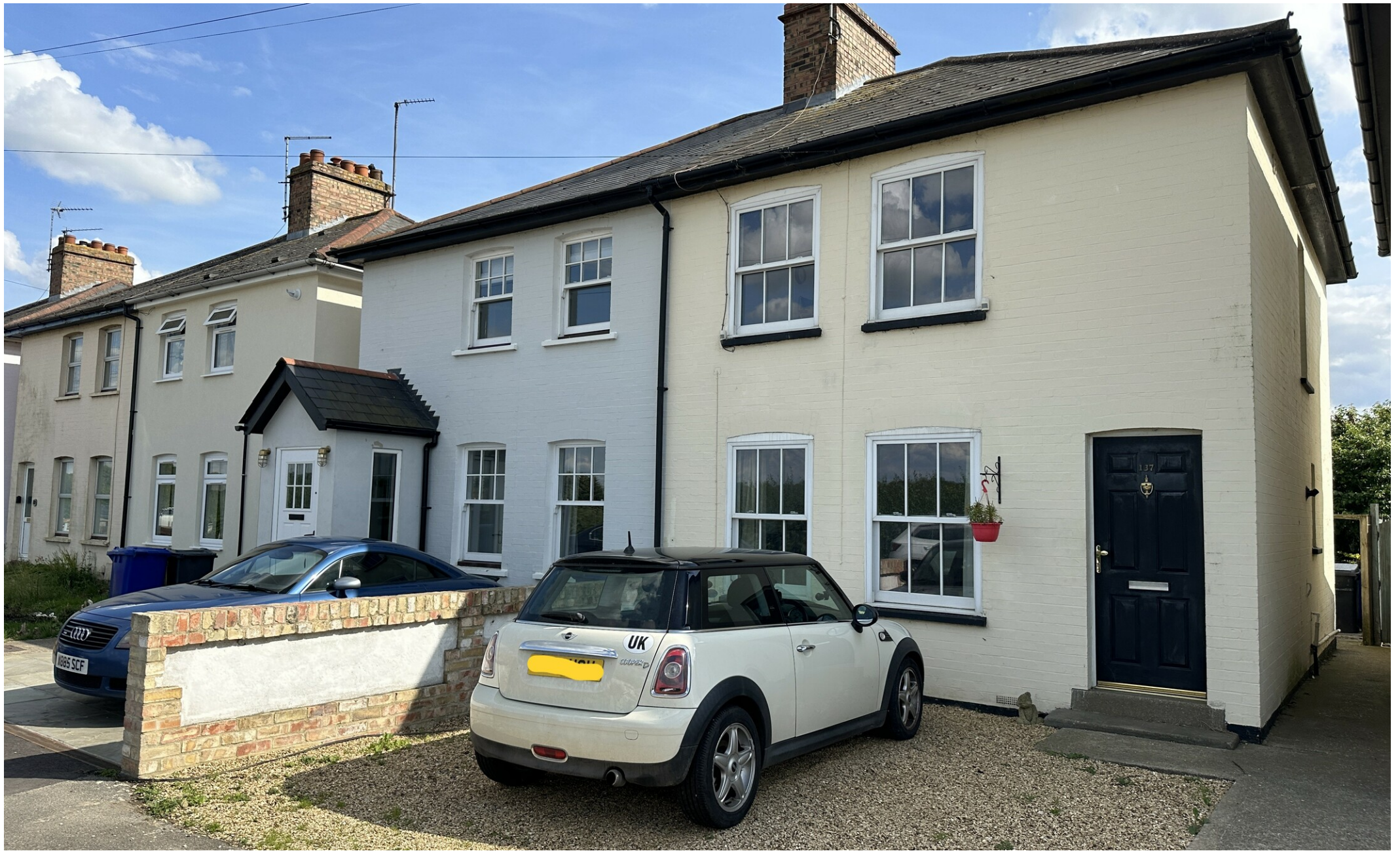
Burwell Road, Exning
